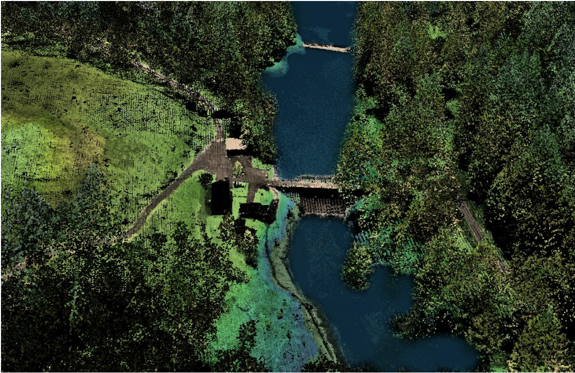
Figure 10. The top image is a 3D point cloud looking north at the Malinowski Dam containing the Aberdeen Reservoir in Grays Harbor County, Washington, colored by height and intensity. The bottom image is a 3D point cloud looking south at the lower part of the Aberdeen Reservoir in Grays Harbor County, Washington, colored by height and intensity.
